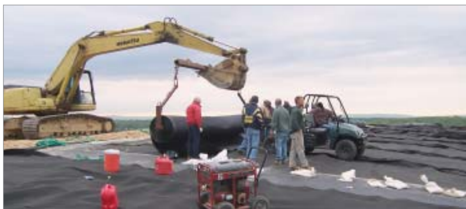
Contractors install the necessary liner at the Berkeley site.
